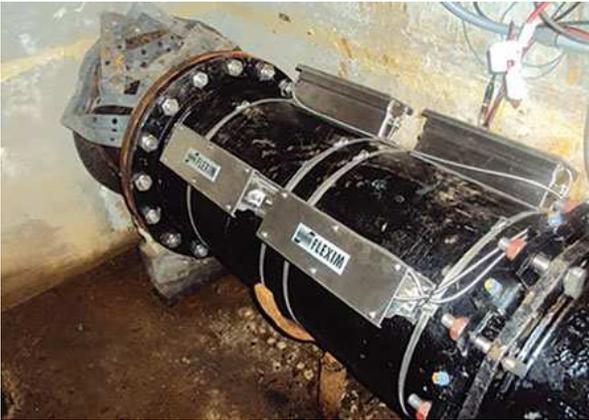
FLEXIM uses a patented permanent coupling pad, so there is no need to take the sensors off the pipe to reapply an ultrasonic couplant.
