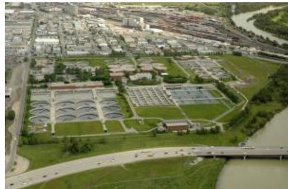
Controlling costs was a primary reason Calgary invested in BNR. Today Bonnybrook (design capacity of 132 mgd) is the largest BNR plant in Canada and the largest cold-weather BNR plant in the world. It treats an average daily flow of 111 mgd, operating 10 state-of-the-art BNR bioreactors that employ biological phosphorus and nitrogen removal processes. Specifically, the plant uses the A<sub>2</sub>O BNR process with return activated sludge nitrification.
