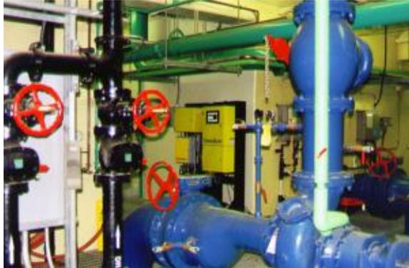
When the analyzer monitoring the final effluent alerts the operators to deterioration in the process, they check the data from the other four analyzers to determine which bioreactor is causing the problem. The analyzers were a significant upgrade from the time-consuming process of grab sampling and lab testing to monitor the bioreactors.
