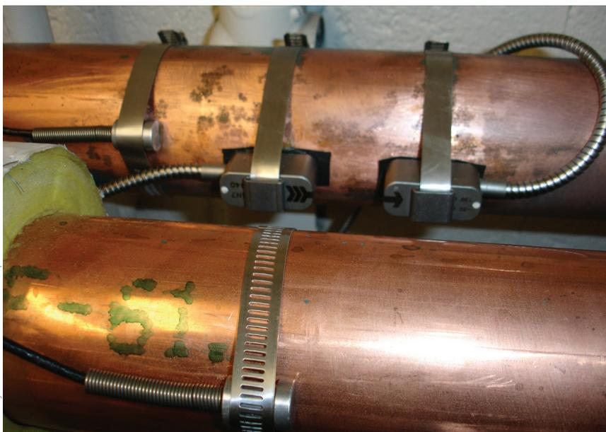
Ultrasonic flow meters are capable of accurately measuring low flows during off hours in a CHP environment.
