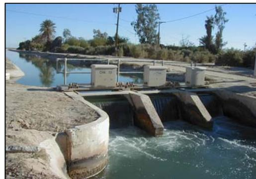
Figure 1 Trifolium 13 Check structure.
